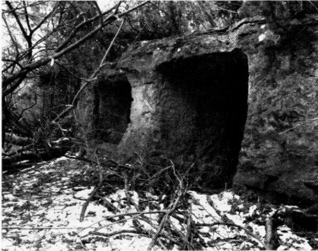
External view to the east in 1987. Note the small thickness of the iron-cemented rock forming a strong roof to the tunnels. Each opening is approx. 2 metres square. Photo by Nick Catford.
